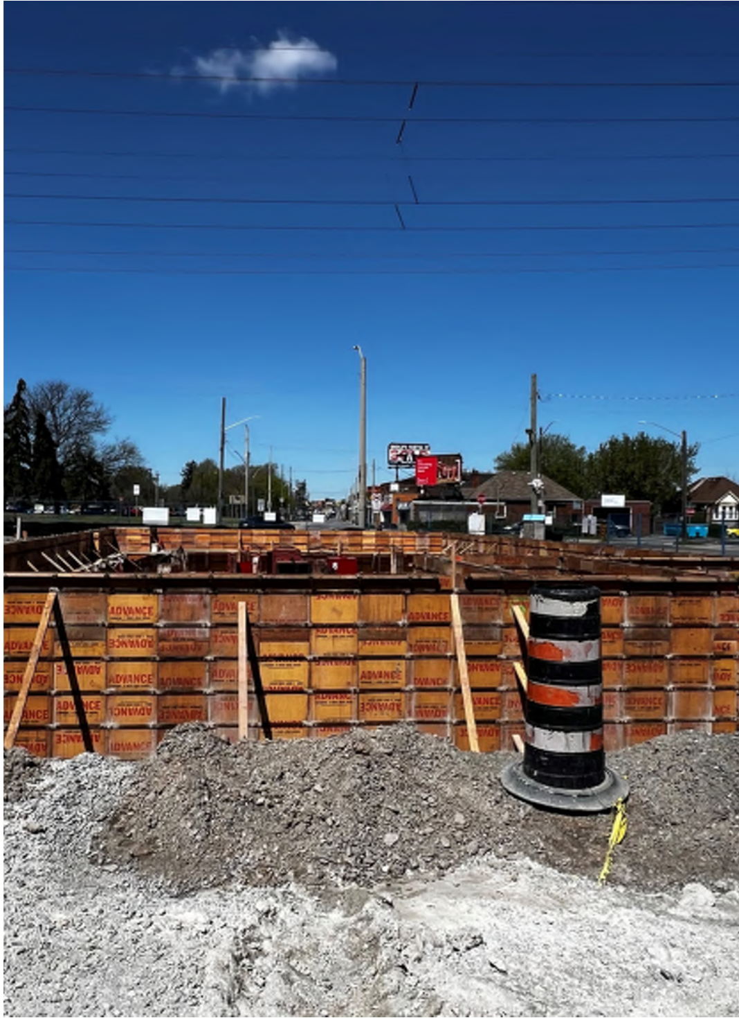
MAY 2 ND 2024 Form-work for Foundations.
