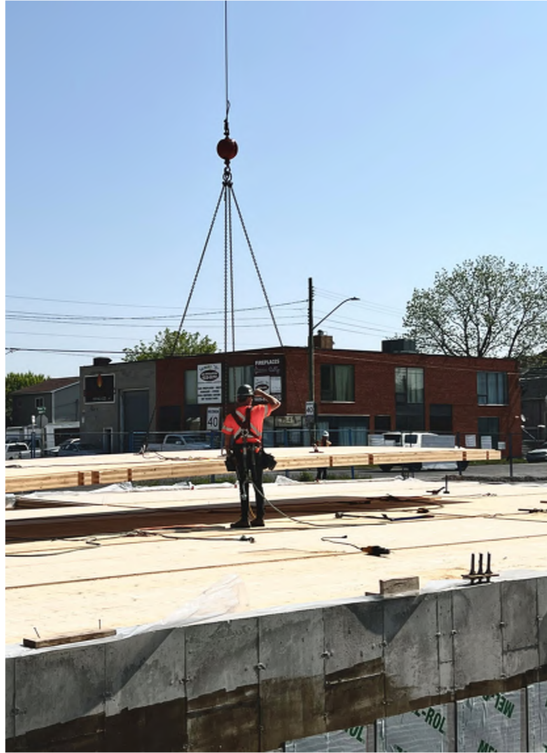
MAY 16 TH 2024 Basement CLT Panels and Ground Floor CLT Panel installation.
